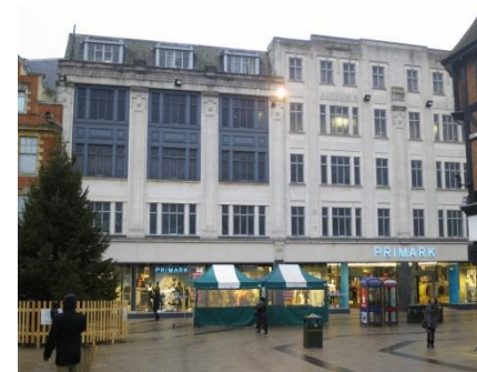
View looking west across Market Square
